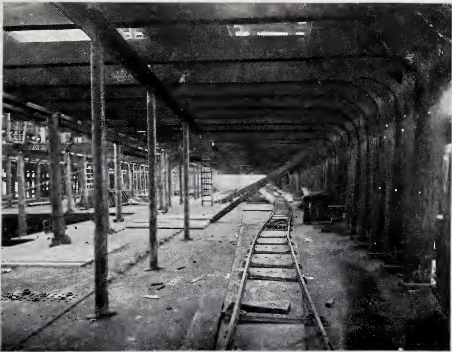
ONE OF THE DECKS OF THE "LUSITANIA" IN COURSE OF CONSTRUCTION.
