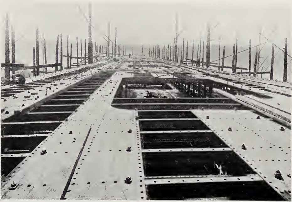
THE SHELTER DECK OF THE "ORSOVA" IN COURSE OF CONSTRUCTION.
